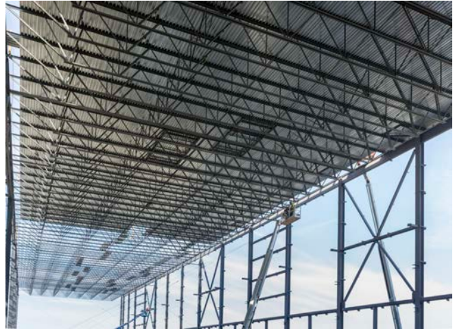
PJC Office – Varennes, QC (Canam Group Inc.)
