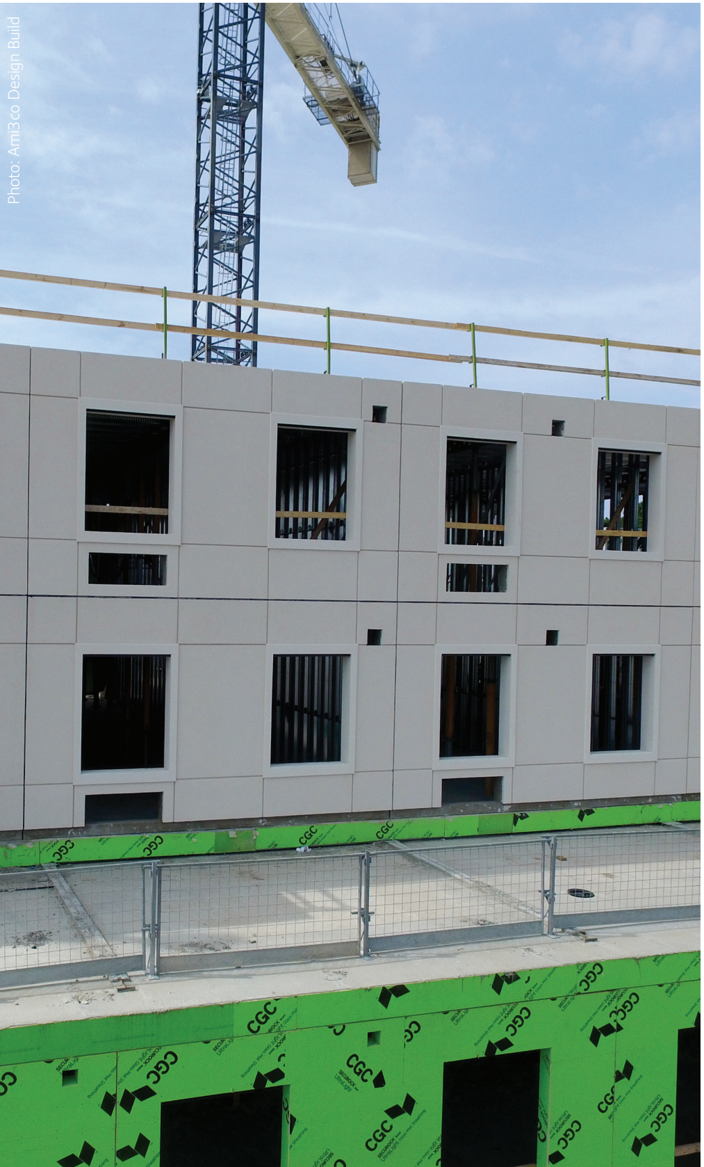
ABOVE: The building envelope is made up of prefabricated and prefinished EIFS (exterior insulation finishing system) and #1 panels using steel stud frame backup.
