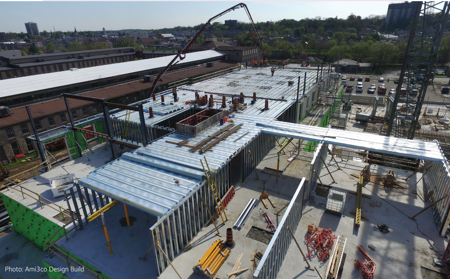
ComSlab® long span floor system prior to concrete being poured showing both wind bearing cold formed steel sections (CFS) and axial-load bearing CFS.
