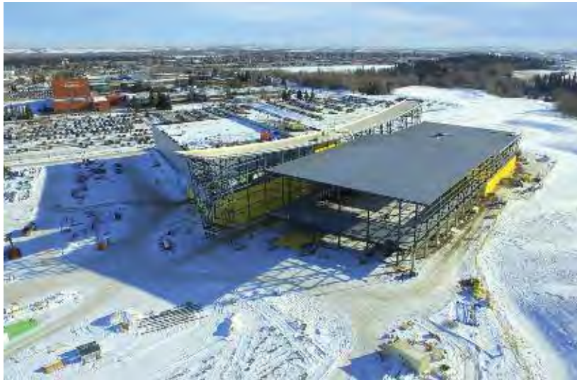
Unfinished arena showing extensive use of load bearing cold formed steel sections on exterior walls.
