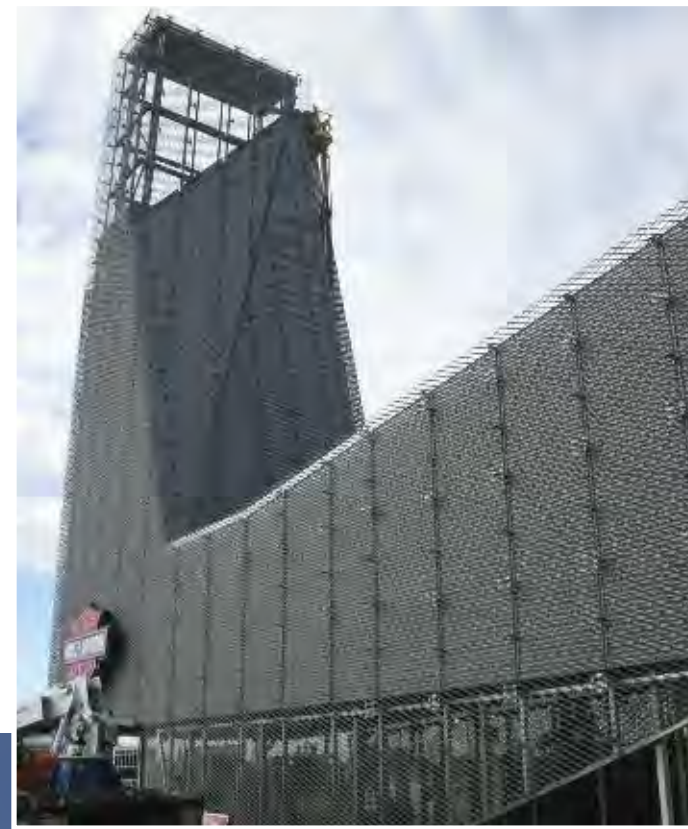
Installing the Galvalume. The top of the tower is left open.
