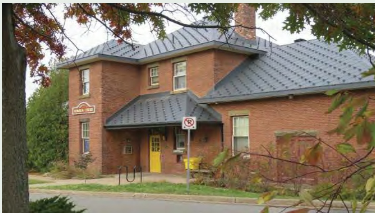
South and Northwest elevations of the re-roofed historic Wolfville Railway Station, now the Wolfville Library, showing the diamond shaped pattern roofing tile made from ArcelorMittal Dofasco's pre-painted .45mm (.0179") AZM150 Galvalume using the Granite Deep Mat paint system coloured QC60036 Graphite Gray, with snow guards.
