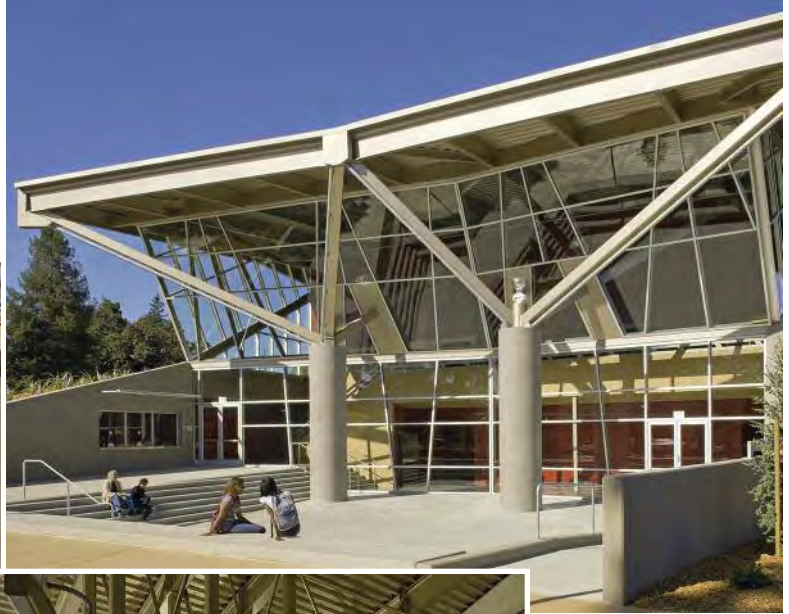
Photograph showing hollow structural steel (HSS) used for the light support framing in lobby area.
