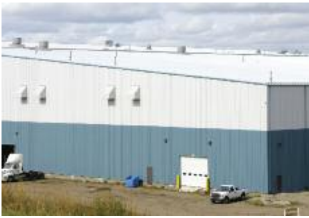
The building's steel standing seam roof is clad with 19,417m 2 (209,000 sq. ft.) of unpainted 61mm (.0239") AZM165 Galvalume Plus, with an acrylic coating.
