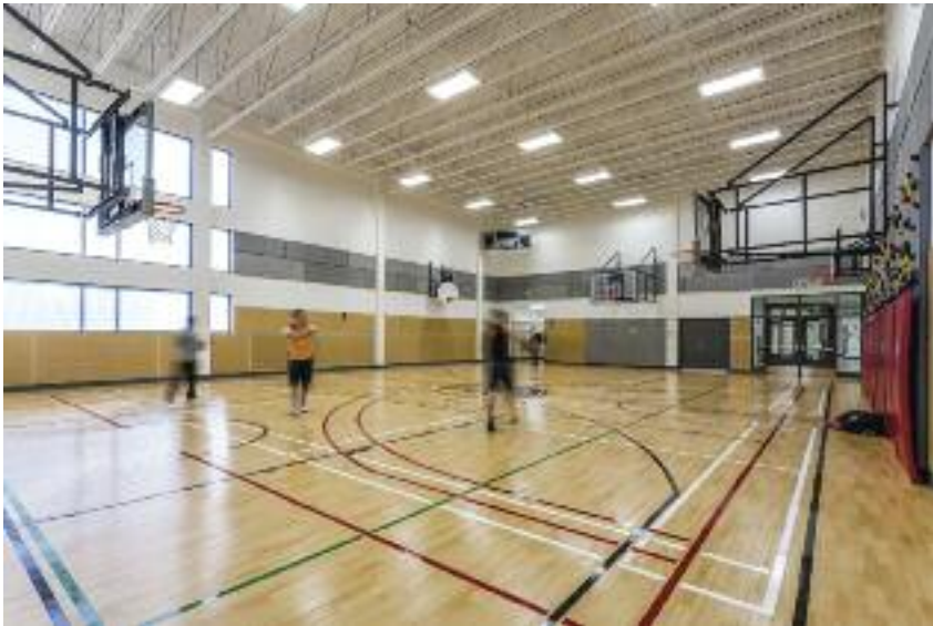
The Field House is a wide span rigid frame pre-engineered steel building. The roof of the steel building system (SBS) housing the soccer field is a “bright white” finish selected to achieve LEED heat island effect credit. The roof also utilizes Behlen’s ‘Thermalguard’ and ‘Vapourguard 32’ systems.
