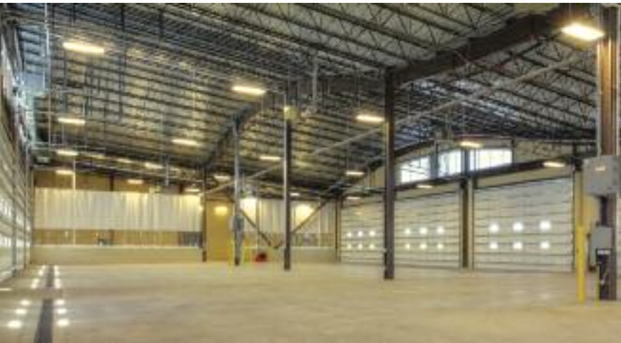
The roof features a crimped steel deck over 660mm (26") deep open-web steel joists supported by a rigid steel frame.
