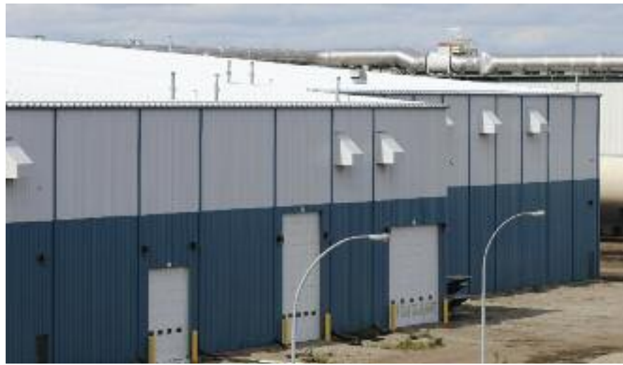
The building's steel standing seam roof is clad with 19,417m 2 (209,000 sq. ft.) of unpainted 61mm (.0239") AZM165 Galvalume Plus, with an acrylic coating.
