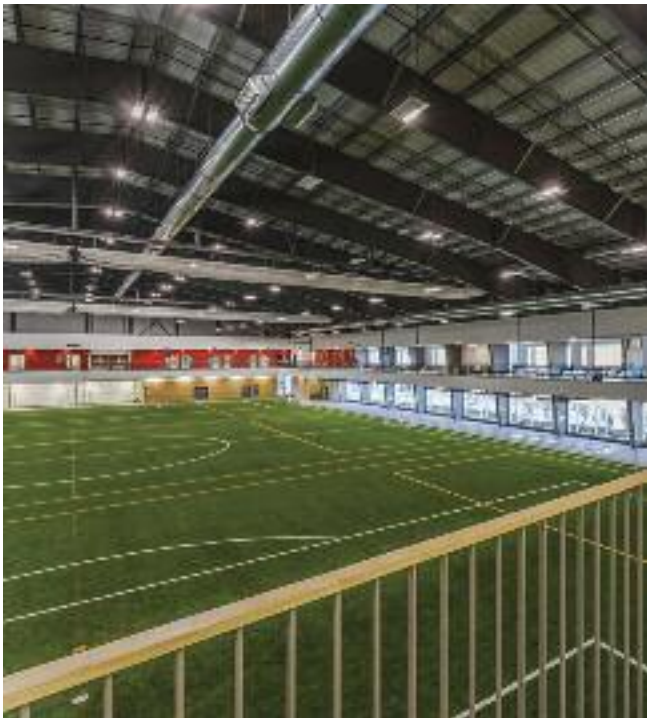
The Field House is a wide span rigid frame pre-engineered steel building. The roof of the steel building system (SBS) housing the soccer field is a “bright white” finish selected to achieve LEED heat island effect credit. The roof also utilizes Behlen’s ‘Thermalguard’ and ‘Vapourguard 32’ systems.
