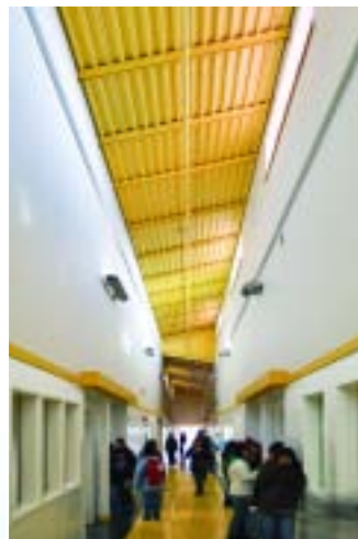
View down the west Middle Years wing, showing the brightly post painted galvanized steel deck.
