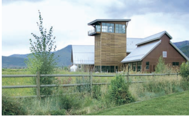
The Galvalume steel standing seam roof contributes to the project's sustainability.
