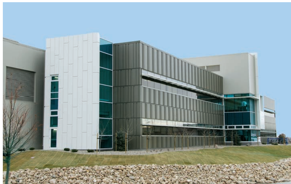
Prepainted galvanized steel cladding used on the two side wings of the building in the 10000 Series paint system coloured QC 2899 Medium Bronze Metallic and QC203 Bone White in four different profiles.
