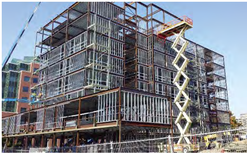
Light steel framing was used for the exterior walls as well as throughout the interior.
