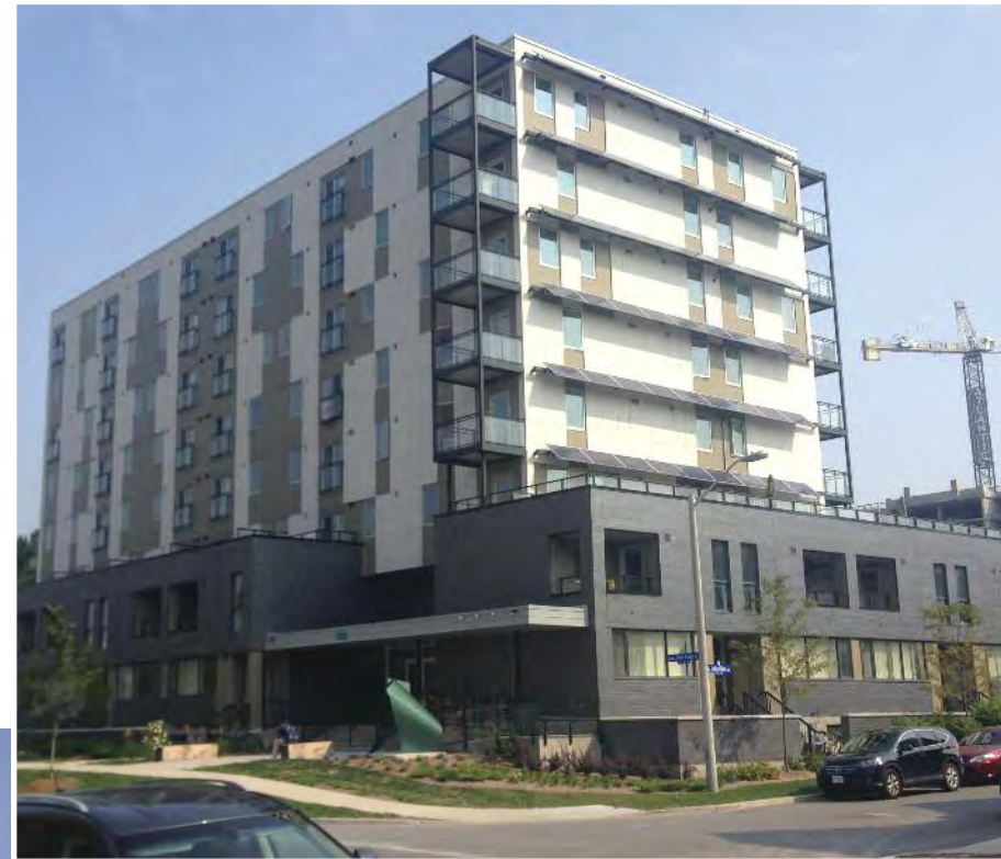
Ottawa is in a Seismic moderate to severe zone. Gerry Morin added, "Steel provides the strength with reduced weight – which is a big advantage in non-combustible construction here."
