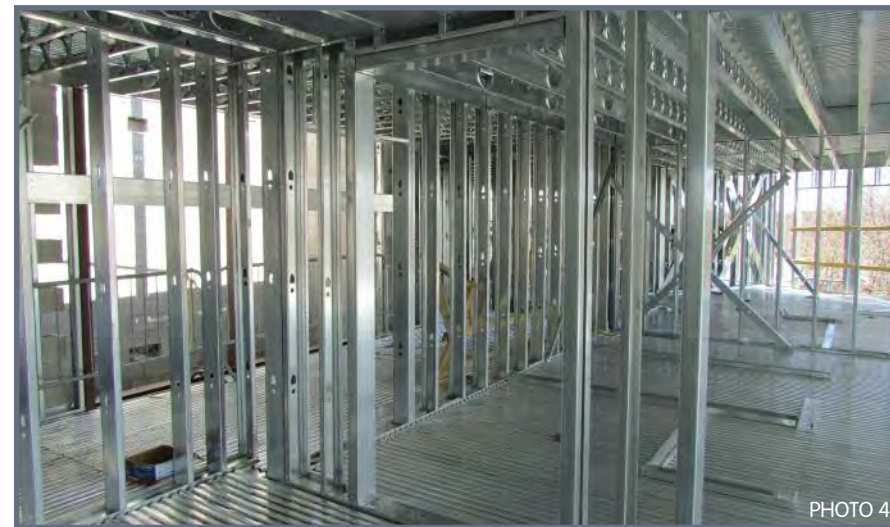
Photo 2: Construction of Cold-Formed Steel Test Assembly
