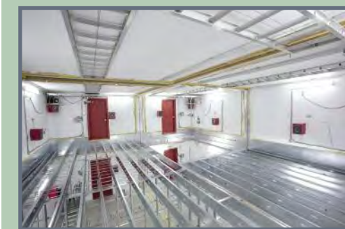
Photo 2: Construction of Cold-Formed Steel Test Assembly
