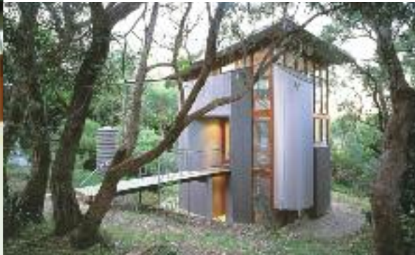
Front View, showing the bridge access to the main living area on the mid-level.
