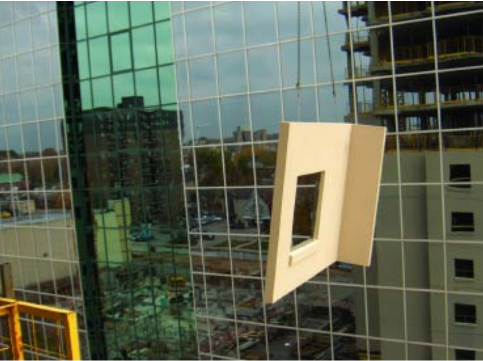
Pre-assembled light steel panels assemblies with a Terraneo finish (dryvit) are easily transported to the site and hoisted in place with simple equipment.
