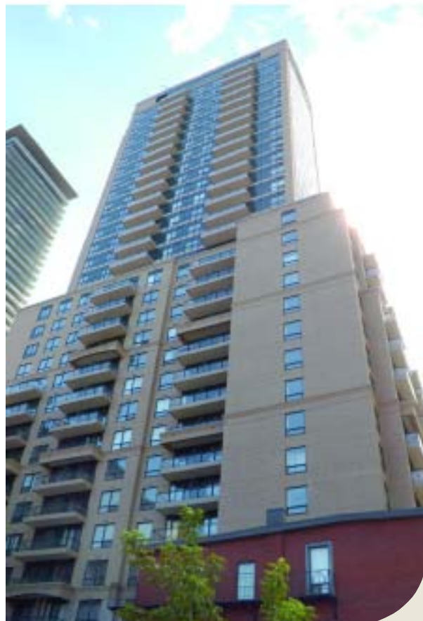
Pre-assembled light steel panels assemblies with a Terraneo finish (dryvit) are easily transported to the site and hoisted in place with simple equipment.
