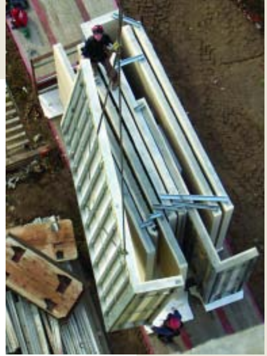
Pre-assembled light steel panels assemblies with a Terraneo finish (dryvit) are easily transported to the site and hoisted in place with simple equipment.
